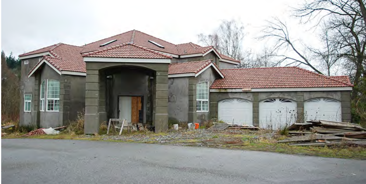
Figure 12.1 Impact of the Great Recession The impact of the Great Recession can be seen in many areas of the economy that impact our daily lives. One of the most visible signs can be seen in the housing market where many homes and other buildings are abandoned, including ones that midway through construction. (Credit: modification of work by A McLin/Flickr Creative Commons)
