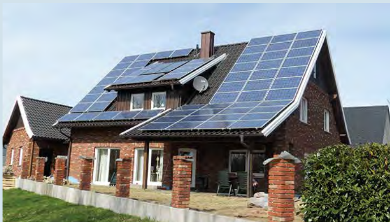
Figure 4.9 Although solar panels can reduce your carbon footprint, the tiles are much more expensive than standard roofing tiles. (credit: "Typical Solar Installation" by Tim Fuller/Flickr, CC BY 2.0)
